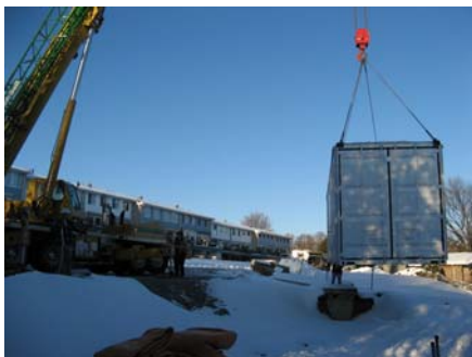
Loading of containerized part of the plant in February 2009
