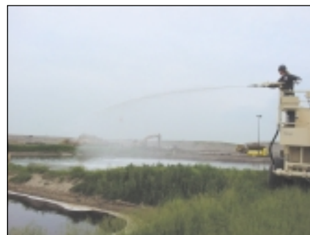
Left: 250 litres of BioStreme concentrate was used to shock each pond.
